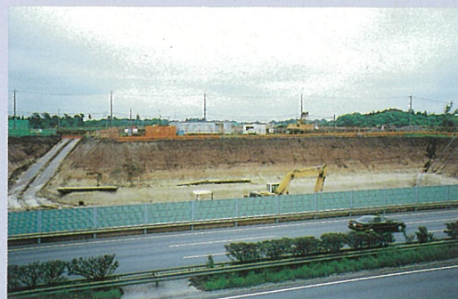
②橋梁下部工事
