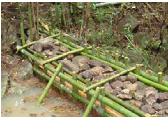
Figure 3 Rock-bamboo check dam
