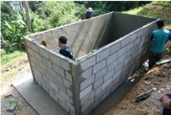
Figure 2 Concrete water storage
