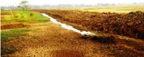
Fig.1: Renovation of canal & de-siltation work
